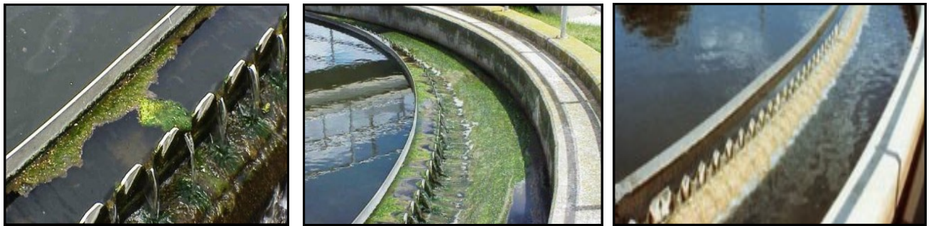
Pictures below showing before and after installing ASMP1000.A in Clarifier
